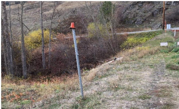
Photo 1: Dam safety signage missing from east abutment – requires replacement.
