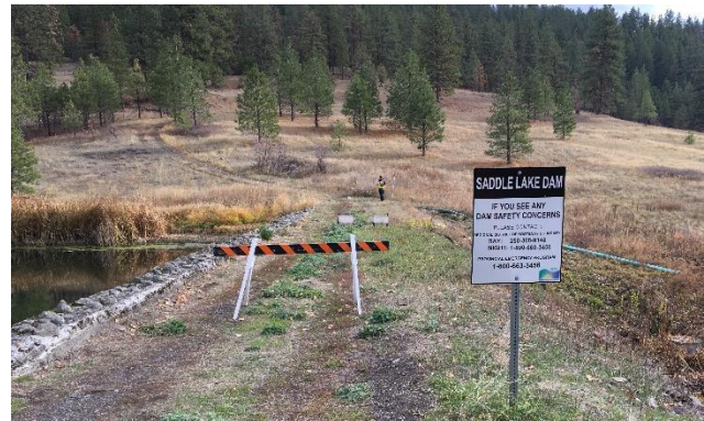
Photo 2: Small barriers on dam crest to deter vehicle traffic, and intact dam safety signage on west abutment.
