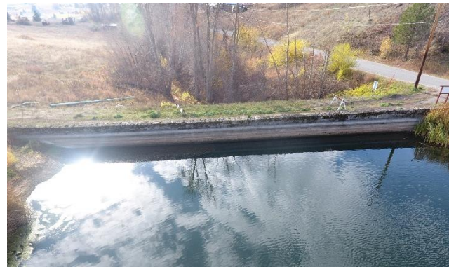
Photo 4: View of the concrete face of the dam.
