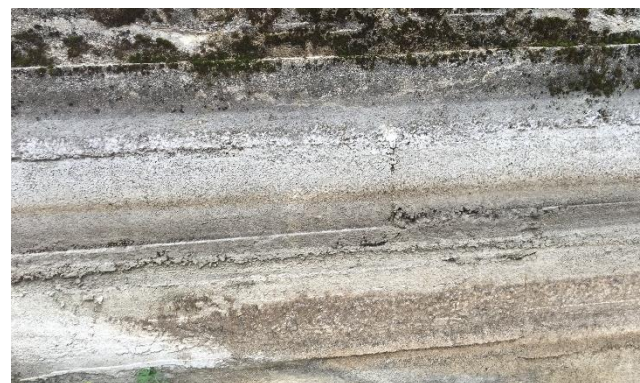
Photo 6: Upstream concrete face in generally good condition; consider patching concrete to extend the life of the dam.
